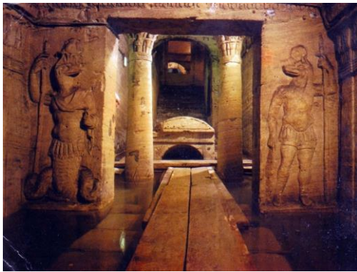
Figure 1. Catacomb of Kom al-Shokafa catacomb with wastewater on the ground.
